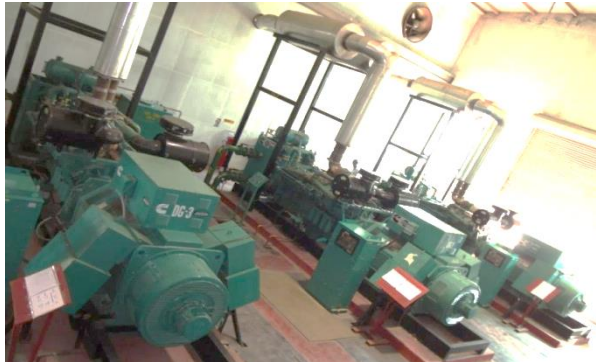
Generators Coupled to Cummins Engines
