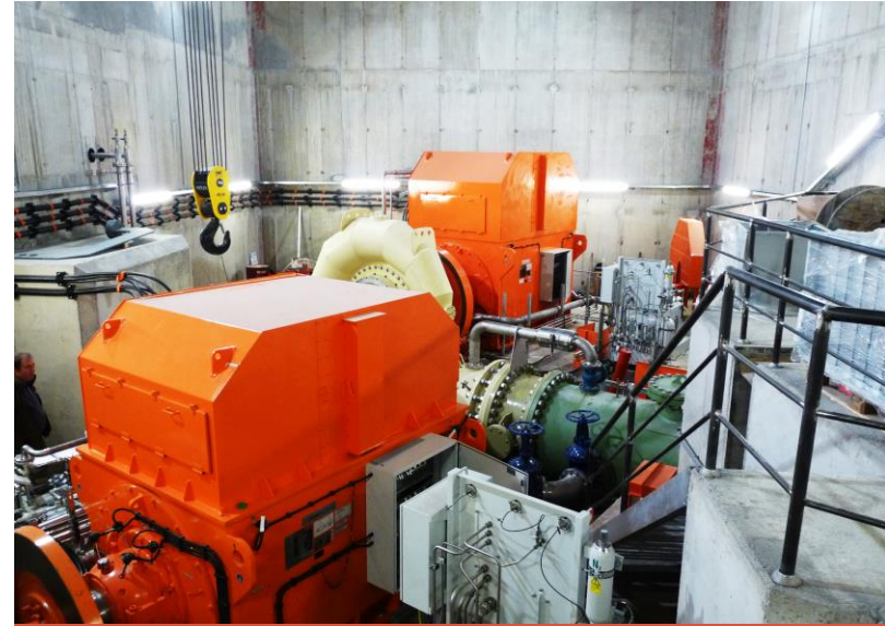
10.16MW & 4.93MW Generators – DECAN Project – Kosovo - KELAG
