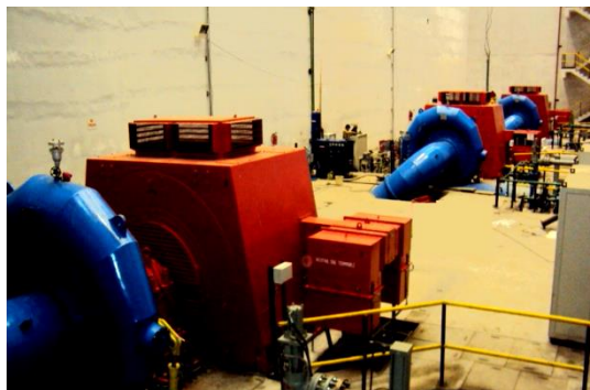
10.64MW Generator - BHILANGANA Project
