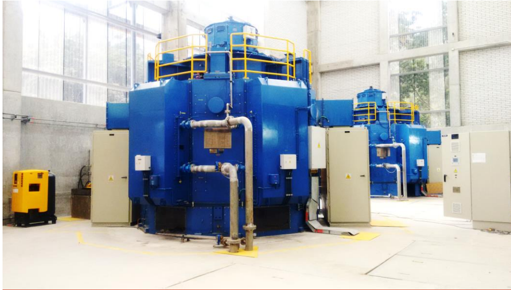
30MVA Generators – San Miguel - Colombia
