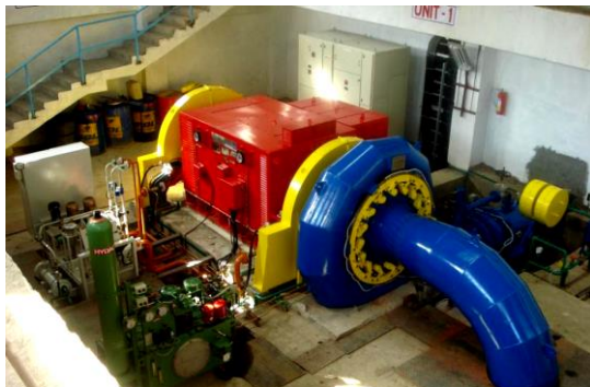
1.75MW Generator - SUBHASH Project
