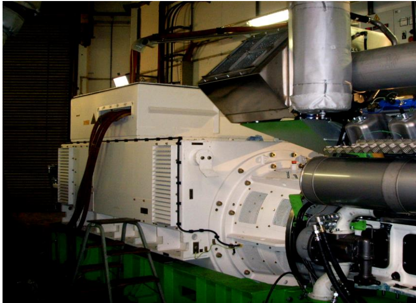
GE-J 620 Series- Coupled to 4.5MVA GEJ Gas Engine
