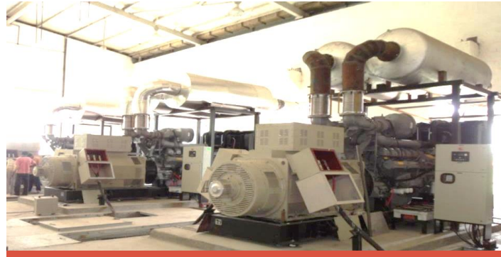
Generators Coupled to Perkins Engines
