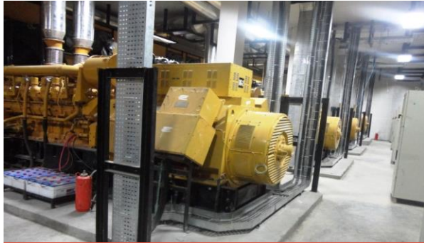
Generators Coupled to CAT Engines
