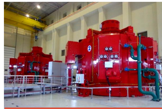
23MW Generator - CAMBASI HEP, TURKEY
