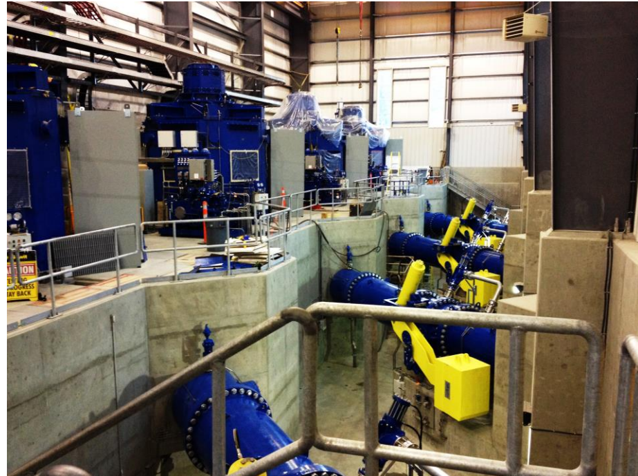
12.159MW Generators - KOKISH Project - Canada
