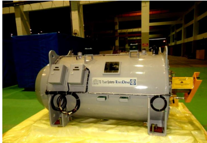
2MW, 1440rpm – Synchronous generator
